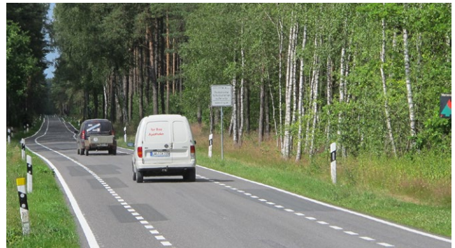
Pilot project: cycle lane on a rural road in the Landkreis Ludwigslust-Parchim (Mecklenburg-West Pommern). © Urbanus GbR
