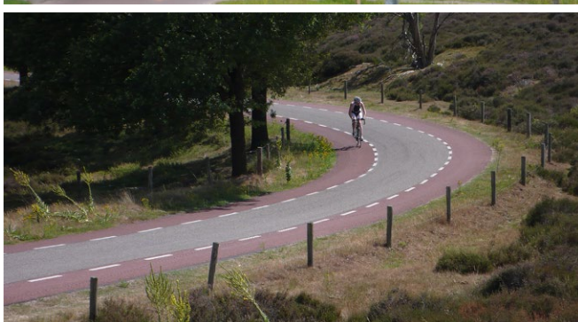
Dutch impressions, from top to bottom: Traffic-calming junction design in the province of Friesland; 60km/h (37 mph) rural road in the province of Friesland; cycling facilities indicated by road markings near Nijmegen
