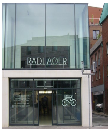
The newly built bicycle garage in the centre of Münster © Westfälische Bauindustrie GmbH
